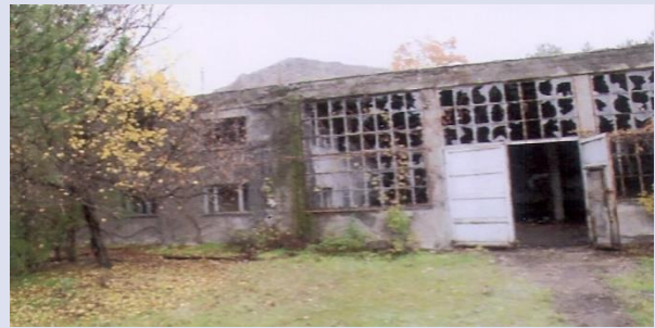
Picture 15. Heating Centre.
